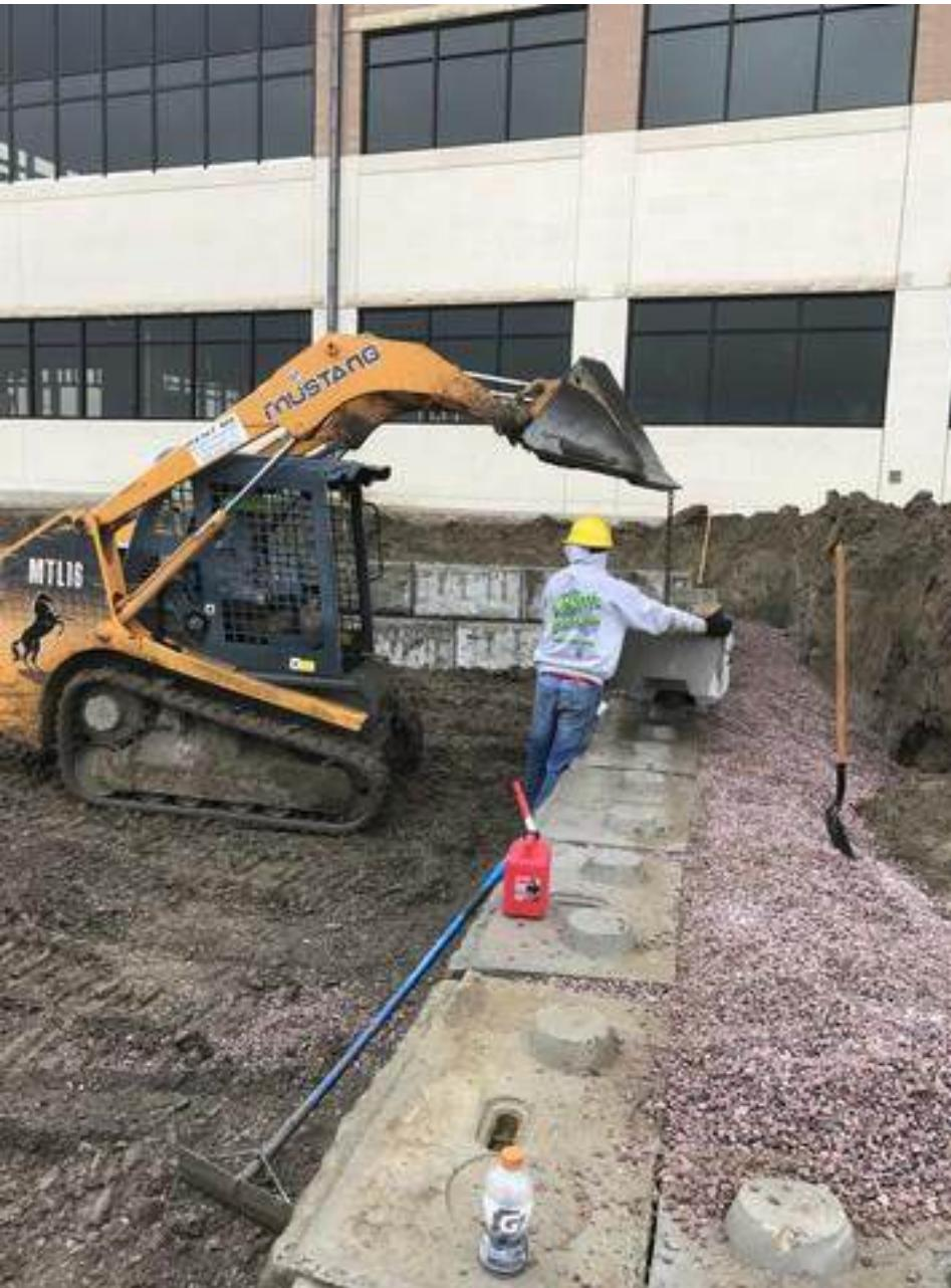
Use crushed rock for backfill this allows drainage thru the wall.
