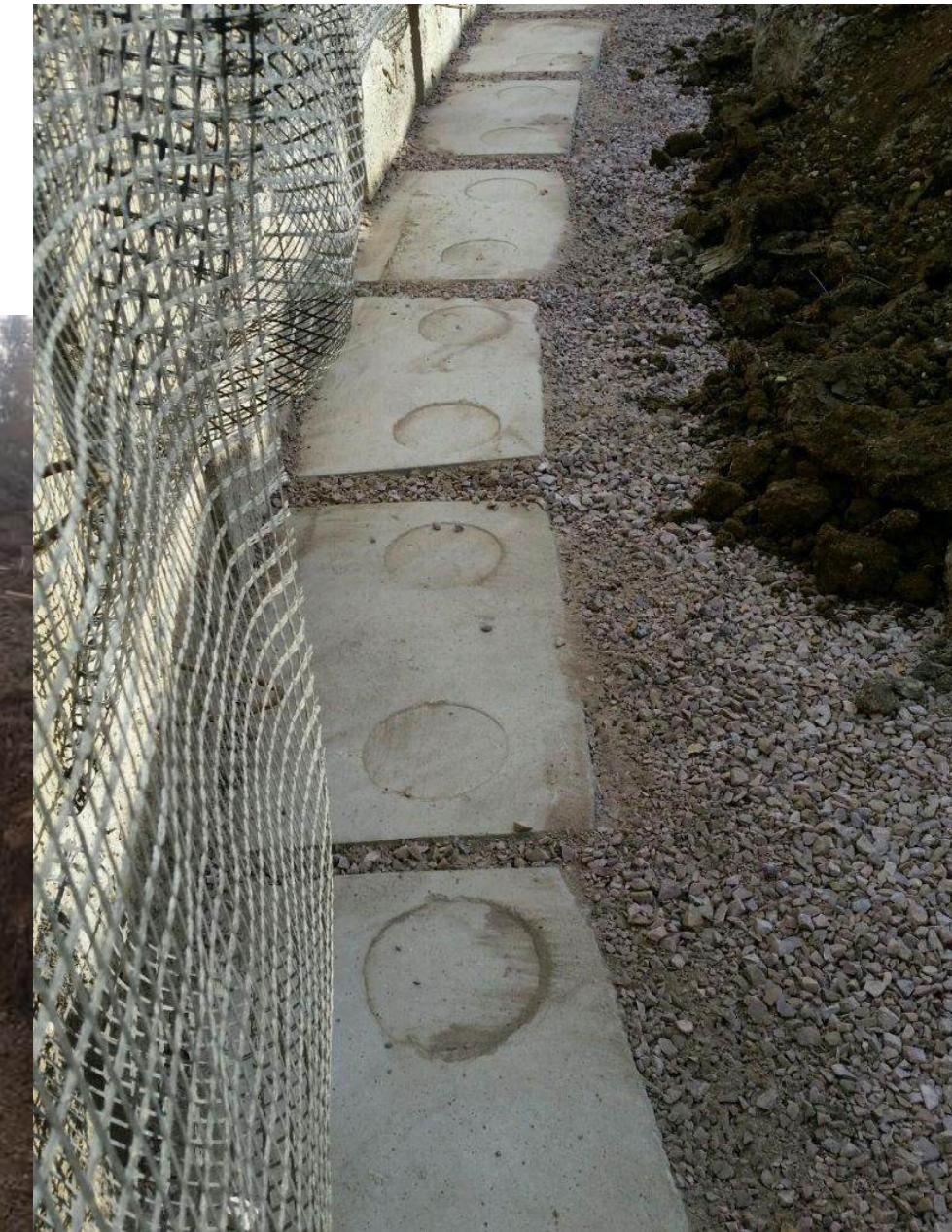
Compact your 6-8" base of gravel or crushed concrete with a packer then you can start placing your base blocks. If you are going over 8' high I would recommend using our 4400# base blocks. They will give you an excellent foundation for placing the rest of the blocks on. You may have to use more than one row of base blocks depending on your soil and height of your wall. You can also use geogrid to reinforce your wall or use a combination of both depending on your situation.
